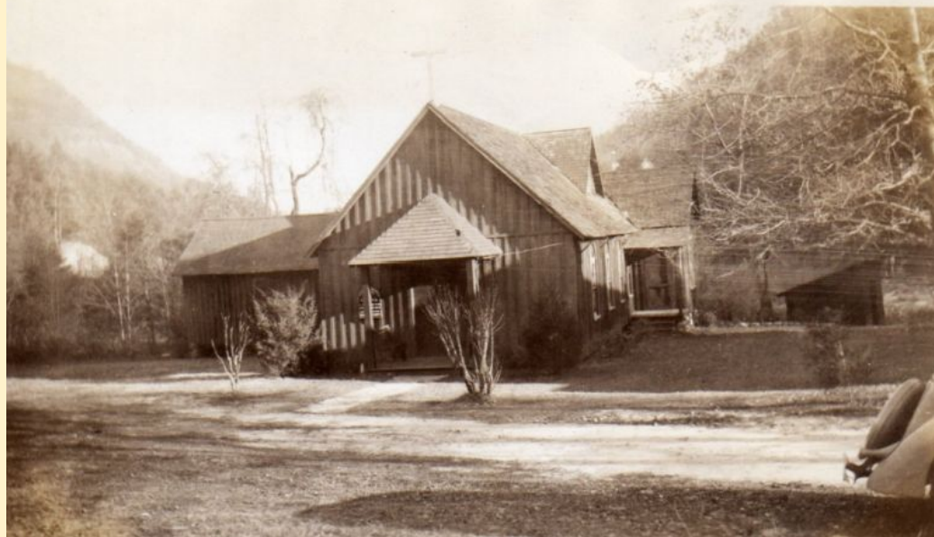
The remodeled church building on the River where the Hickory Nut Creek joins the Rocky Broad, (present location of the Bat Cave Fire station.)
